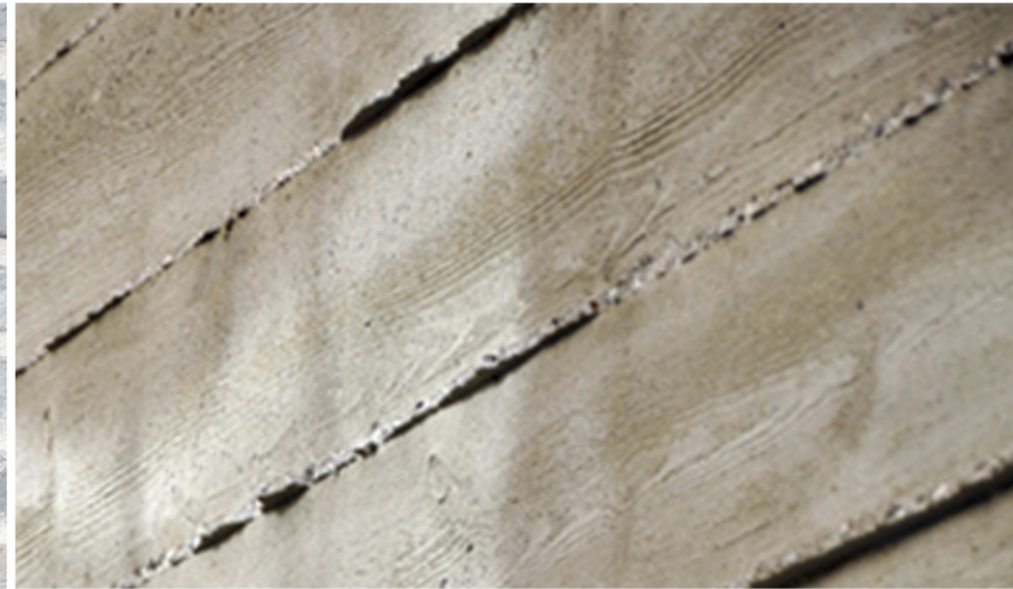
BOARD FORM CONCRETE
